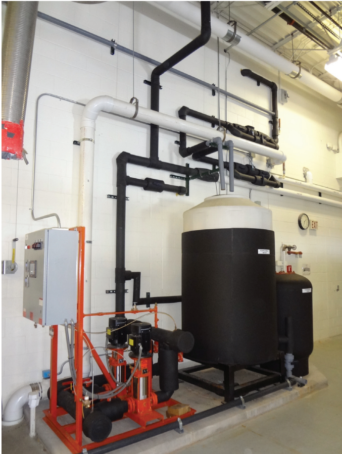
Water reuse system location in apparatus bay.
